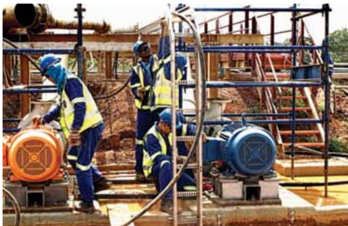
Installation of pumps at one of the solution ponds.
