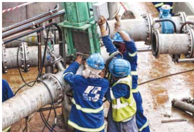
Valve installation
