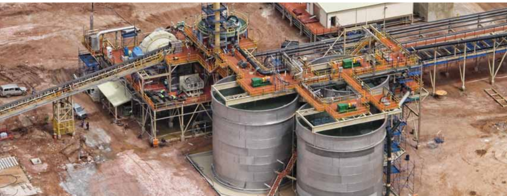
Ball mill and leach tanks — Kinsevere Stage II plant.
